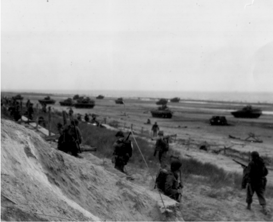
SC-320891: Amphibious DD M4A1s from the 70th Tank Battalion sit on Utah Beach on 6 June 1944. The Allies used DD tanks in Operations Overlord and Dragoon and in the Rhine crossing. (Signal Corps photo)
