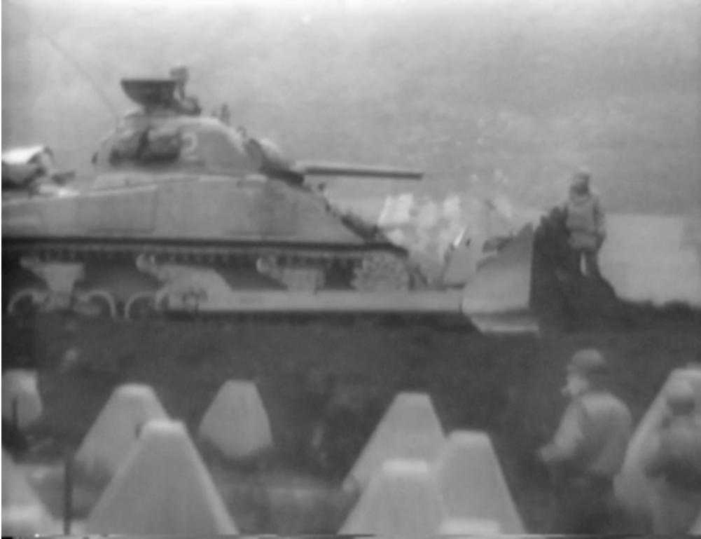
111-HRB-30_5: Taking their cue from German farmers, engineers use a tank-dozer to create a road across the dragon's teeth. (National Archives, Signal Corps film)
