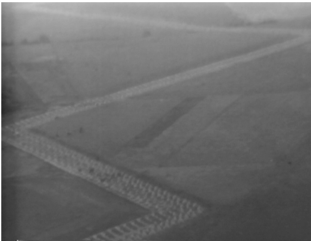
111-HRB-30_4: An aerial view of Siegfried Line or West Wall dragon's teeth near Aachen, Germany. (National Archives, Signal Corps film)
