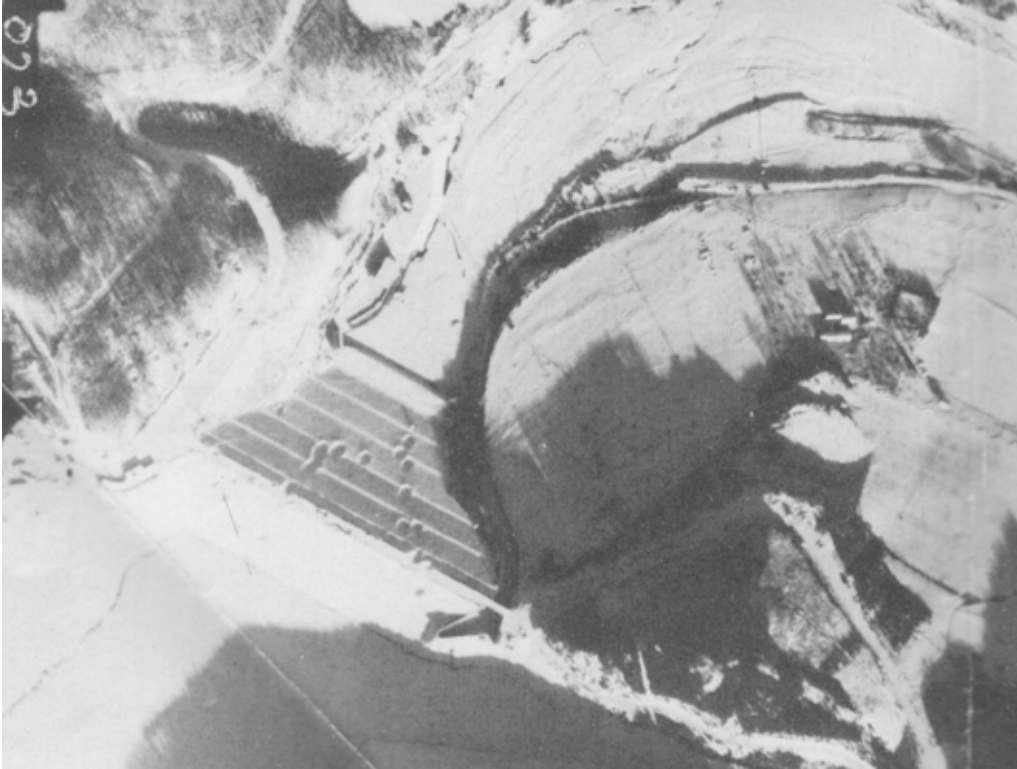
78thID_3: Aerial view of the Schwammenauel Dam issued to the 78th Infantry Division. Cratering from bombing raids is visible on the dam's face. (National Archives, Signal Corps photo)
