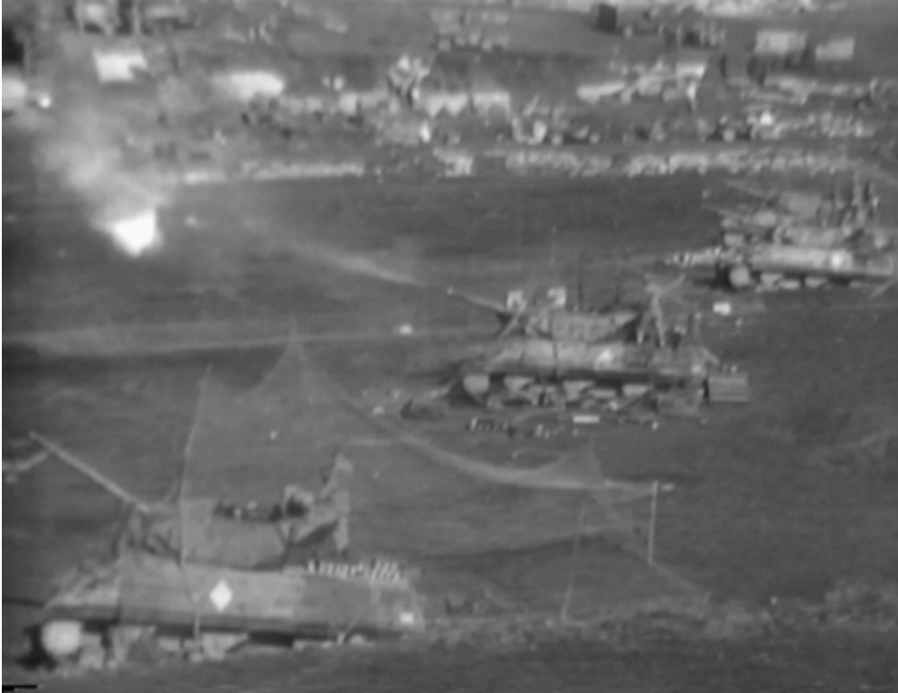
111-CR-1_4: 636th Tank Destroyer Battalion guns shell San Pietro, Italy, before the bloody infantry assault on the town in late November 1943. The mountainous terrain—which started just behind the Salerno beachhead—often relegated the TDs to artillery roles. (National Archives, Signal Corps film)
