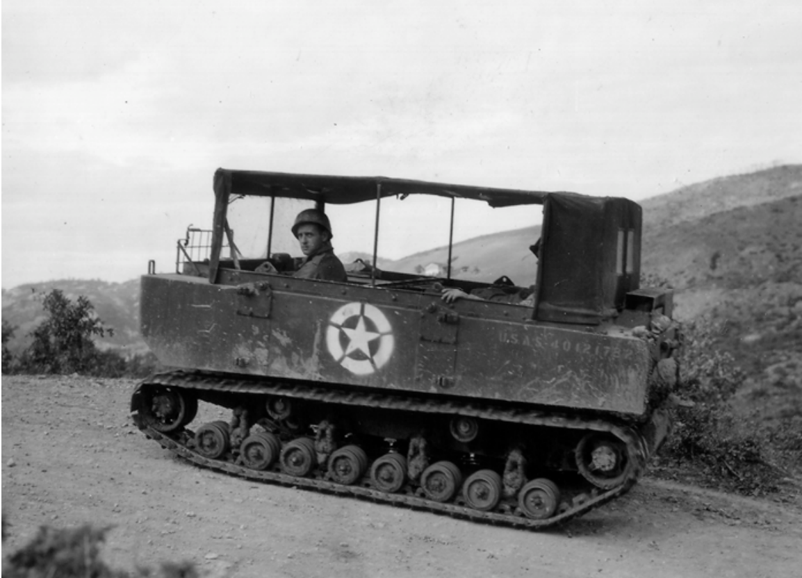
SC-196135-S: The M29 light cargo carrier, known as the Weasel, was not standard issue but served with some battalions in the Pacific Theater. (NARA, Signal Corps photo)
