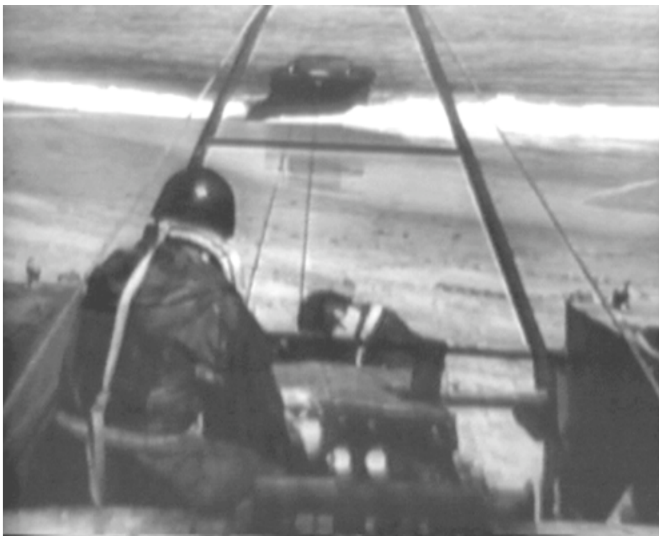
111-CB-60_5: The rear winch on an LVT retriever pulls a disabled amtrac from the surf. (NARA, U.S. Army film)
