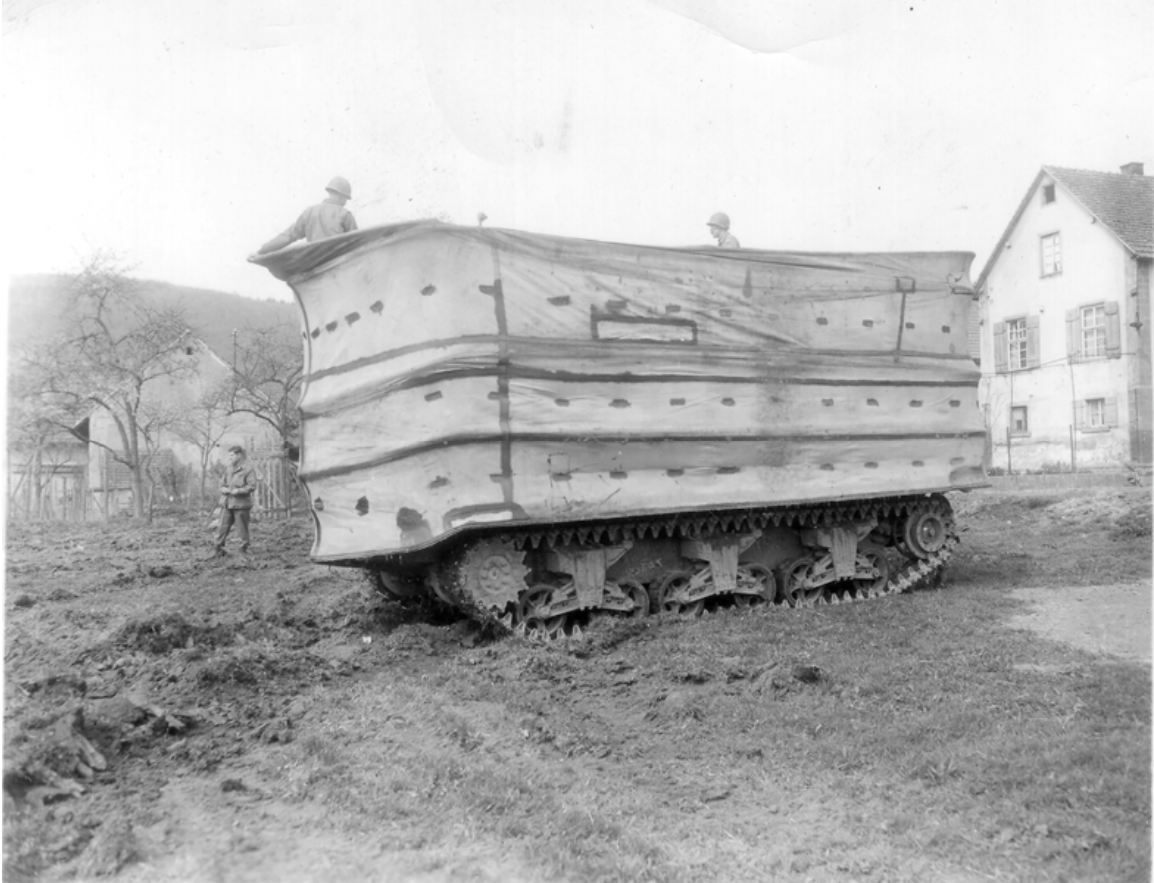
SC-243899: A DD Sherman with screens raised. The commander could steer in the water using a long handle that controlled the orientation of the propellers, as could the driver in response to commands—as he could see nothing! (NARA, Signal Corps photo)
