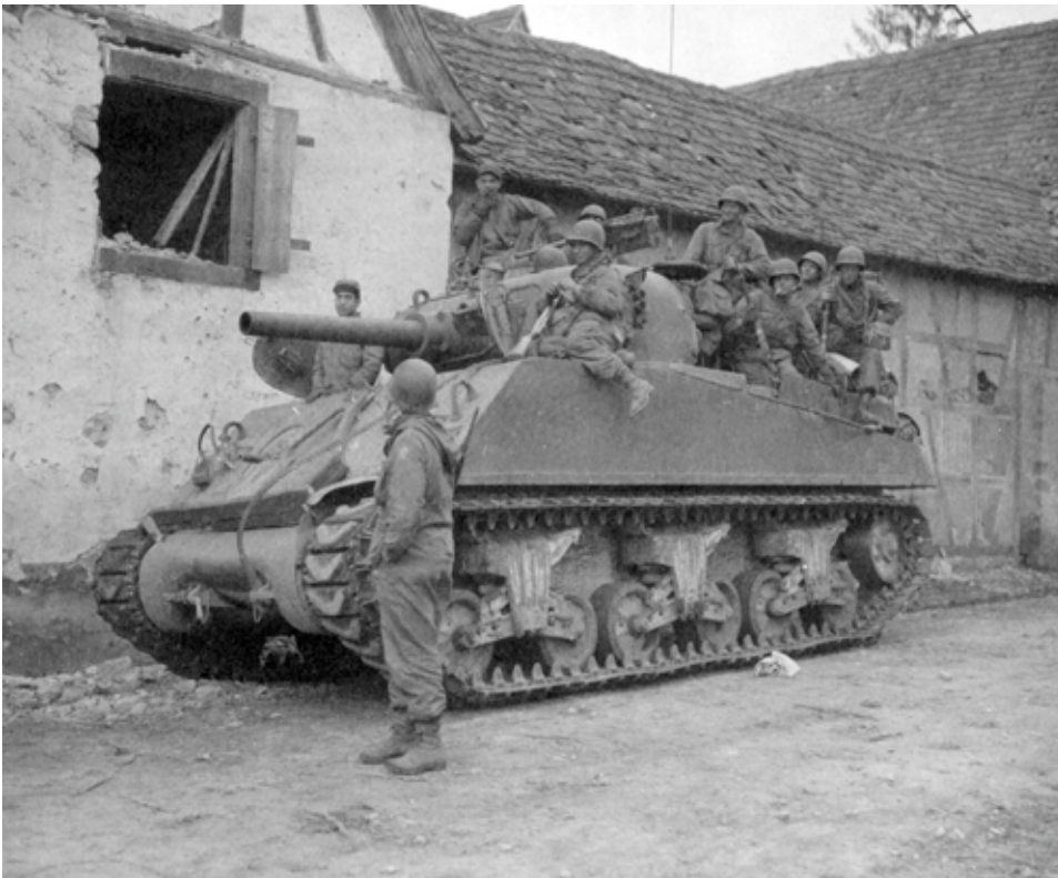
SC-337939: This 105mm assault gun has the 47-degree glacis, which both eliminated the shot traps and provided bigger hatches to the driver and bog. (NARA, Signal Corps photo)
