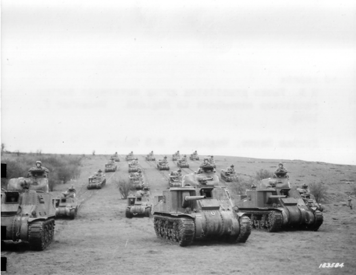
SC-163584: The look of a medium tank battalion under way in December 1942, with more than a company of vehicles visible in this shot. This unidentified separate tank battalion is part of the 1st Tank Group. These are late production M3s, on which the side access doors were eliminated because they weakened the armor protection. (NARA, Signal Corps photo)
